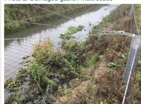
Photo 3: Bank erosion downstream of gabions
