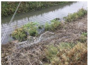
Photo 2: Damaged gabion mattresses
