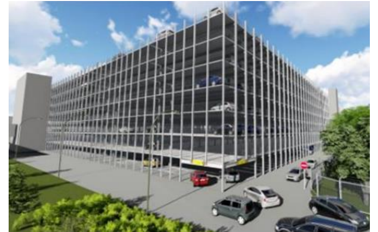
Multi story car park 7
